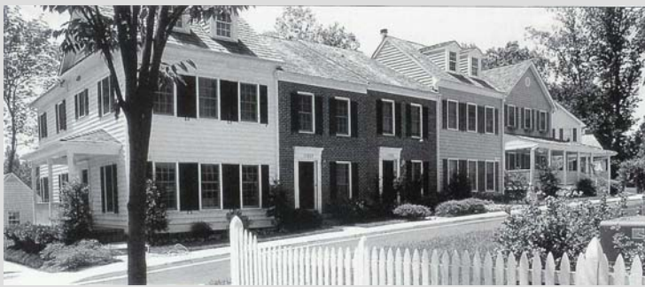
Different siding and roof treatments create visual interest and individualize each unit.
